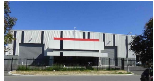
RCWA1 DATA CENTRE PARK
